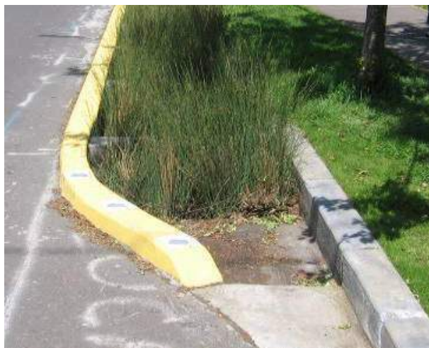
Figure 9-A.3. Stormwater Curb Extensions
